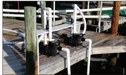
A test ozone treatment system manages the red tide in a canal in Boca Grande, Fla. Mote Marine's ozone treatment system is currently being used to remove Karenia brevis cells and toxins that cause the red tide in seawater.
