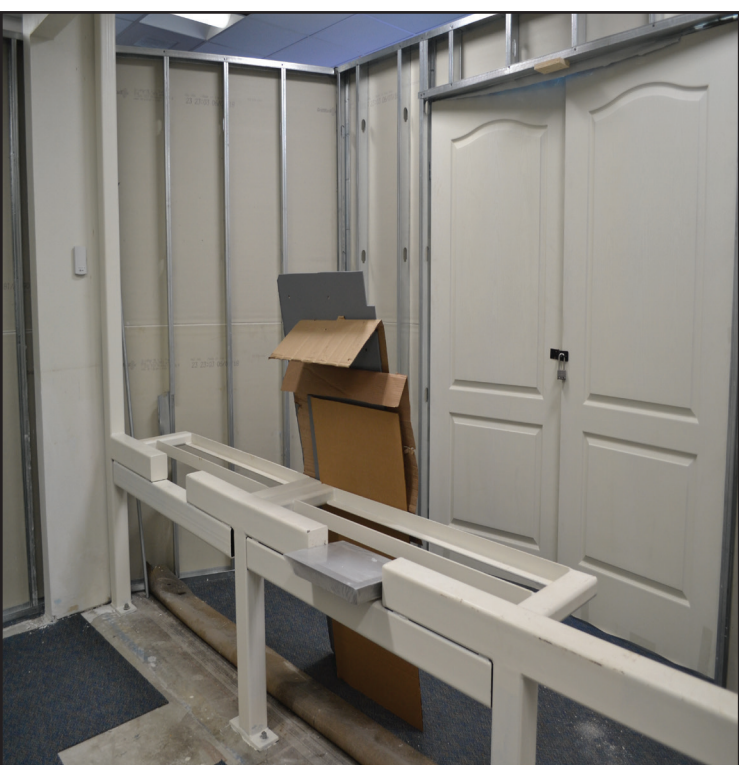
The metal beams seen here, behind the temporary walls used during construction, were installed in order to support the weight of the bulletproof glass. Construction is set to be finished during or shortly after winter break.
