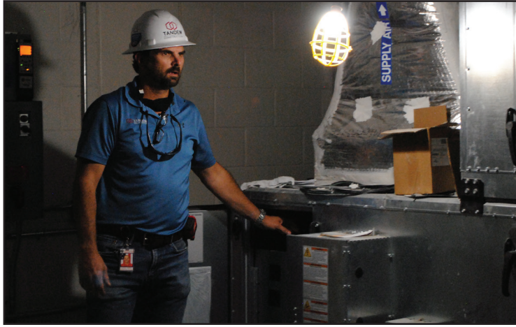
Project manager Nathan Renner stands in front of the new building's air conditioning system. Powered by several chilled air units, the system is specially constructed to prevent outages.
