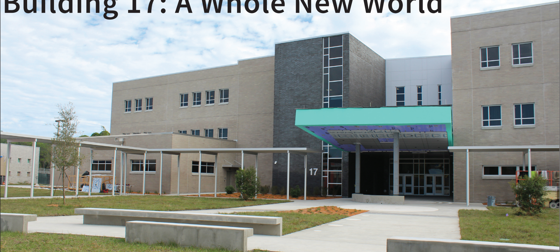
In its final stages of construction, Building 17 gazes across the Pine View campus. The building will be open come second semester. PHOTO BY FELICITY CHANG
