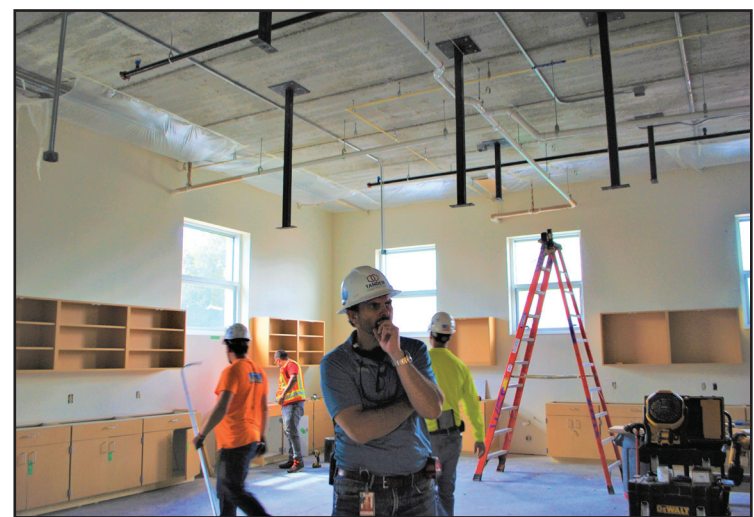
Project manager Nathan Renner looks across a physics classroom during an October tour. The physics rooms’ high ceilings will give students a look at real-life applications. PHOTO BY ALYSON MIZANIN
